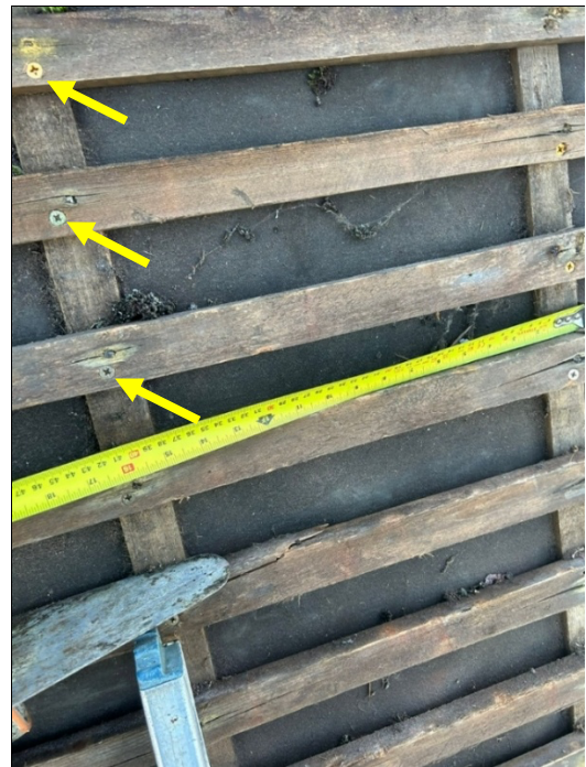
4. Where possible, battens were temporarily resecured with screw fixings. There are also vertical counter-battens with similar age nails.
