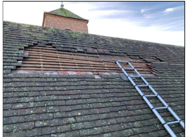
2. Work commenced. Large area of slipped and displaced roofing battens which have slumped onto one another.
